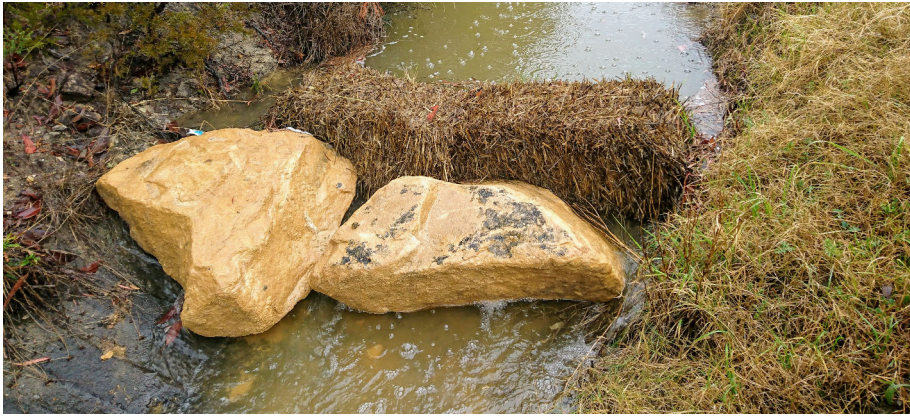
Figure 5.2: Leaky weir in Attunga Creek rock drain. Note the deeper water upstream of the weir.
